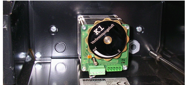
Im. 4: Loosen the mounting bracket including the motor
